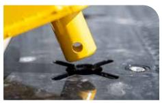
Insert shank into existing keyhole slot on steel deck. If installing on an aluminum deck, see photo 2A.
