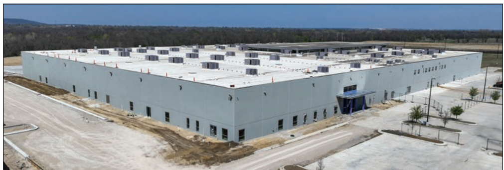
Mohawk Facility (March 23, 2024)
