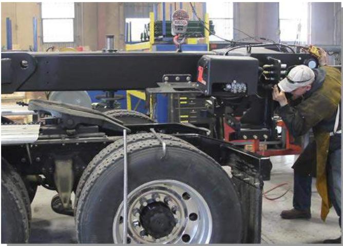
#5) Lower FIFTHWHEELER beam, onto truck locking kingpin into fifth-wheel plate.
