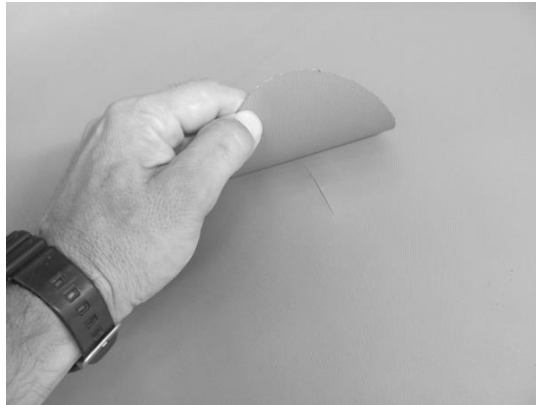
Fig. 2: Choose a correct size of the patch.
