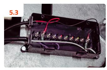
Connect the red wire from the actuator 48" pigtail to a protected power terminal in the junction box and the black wire to ground. **IMPORTANT:** Do not eliminate the provided two-prong quick connector from the actuator pigtail when wiring. Also, wires cannot be reversed to change the direction of operation. The system won't work if the wires are reversed.
