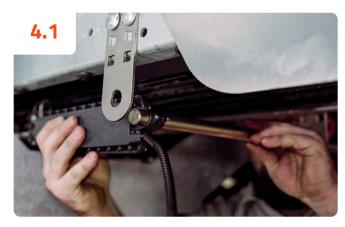
With the wires facing down, slide the actuator(s) onto the actuator mounting bar.
